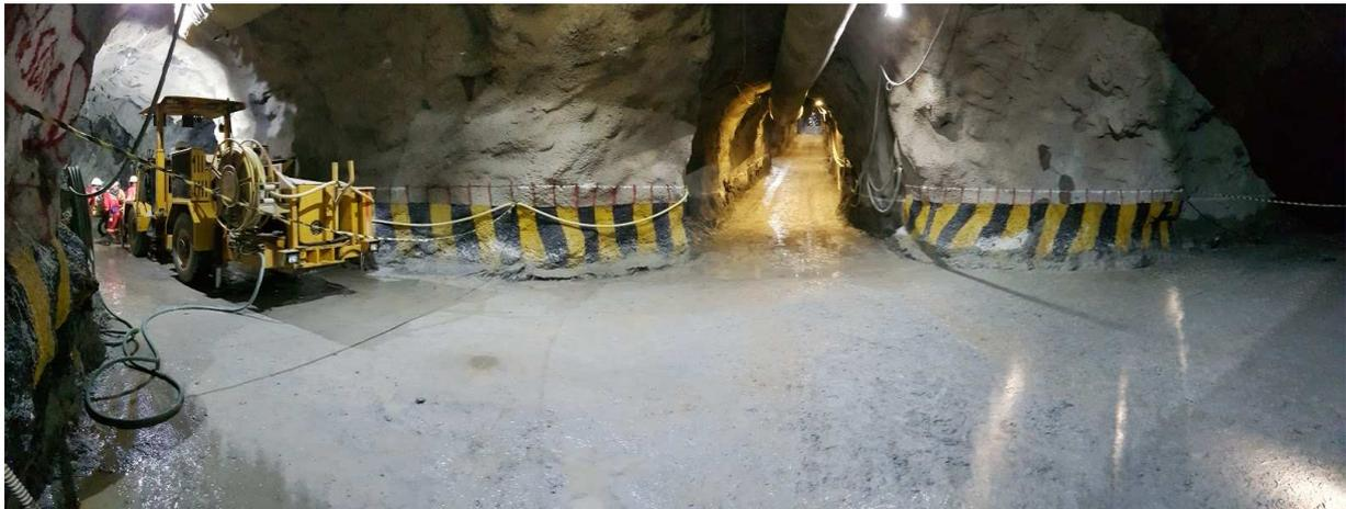
The ore drives are located along the footwall contact of the orebody. These footwall and ore drives extend to the limits of the orebody. Connections between the footwall and ore drives are developed as and when required.
