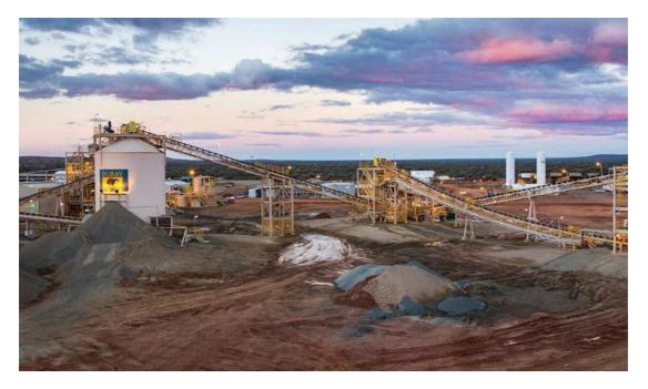
The Andy Well processing facility is a 30,000 tonne per month plant and comprises a two-stage crushing circuit, single stage grinding circuit, gravity recovery circuit and conventional carbon-in-pulp circuit. Commissioned in July 2013, it consistently had above 98% availability and recoveries averaging more than 95% during the final year of operation. Mining at the later stages of the operations was all underground and used the cut and fill method.
