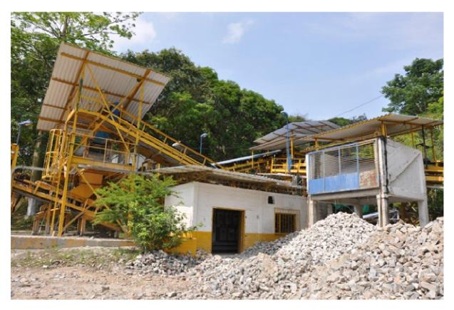
The crushing plant (pictured above) historically operated one shift per day at 10-12 tonnes per hour but has capacity of 20 tonnes per hour, providing sufficient crushed rock to feed the mill. The crushing plant consists of a jaw crusher, cone crusher, vibrating screen and associated belts and bins.
