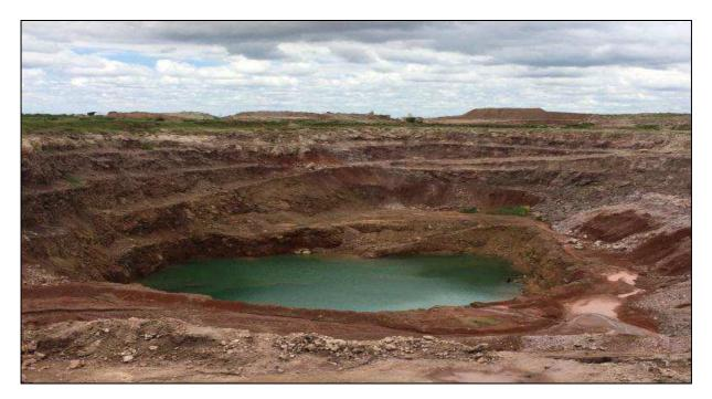
Initial pit design work indicated that approximately 12mn tonnes of kimberlite could be extracted at an average grade of 8 cpht containing circa 900,000 carats. Phase 1 of the BK11 production plant commenced in August 2010.
