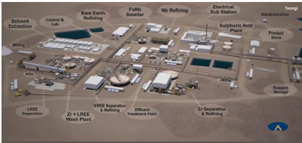
Sulphuric acid used for leaching will be produced on site using a sulphur burning acid plant that also generates electricity and steam for the process plant. A small amount of waste rock will be extracted and transported to a small waste rock emplacement to the southwest of the open cut. The liquid and solid residues from the zirconium processing plant will be transported and stored in liquid residue storage facilities, solid residue storage facilities and salt encapsulation cells.
