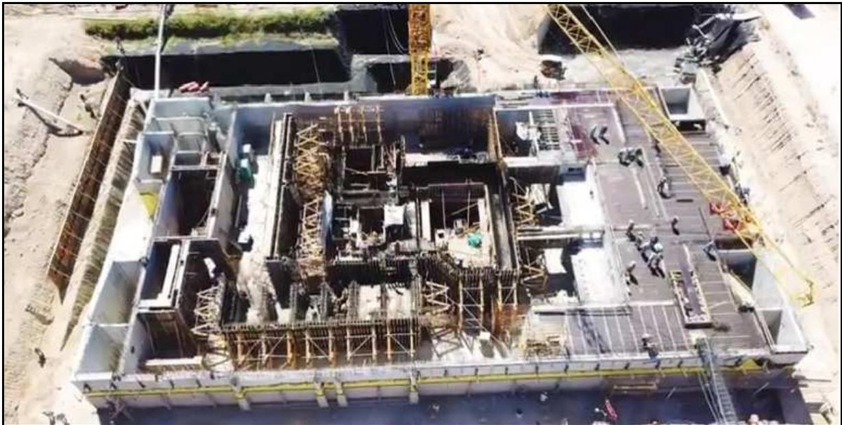
At the Ezeiza Atomic Center, the National Atomic Energy Commission is carrying out the construction of RA-10, the multipurpose reactor with which Argentina seeks to expand current capabilities in the areas of health, industry and scientific research, guarantee the production of radioisotopes of medical use and consolidate its leadership in the nuclear sector.
